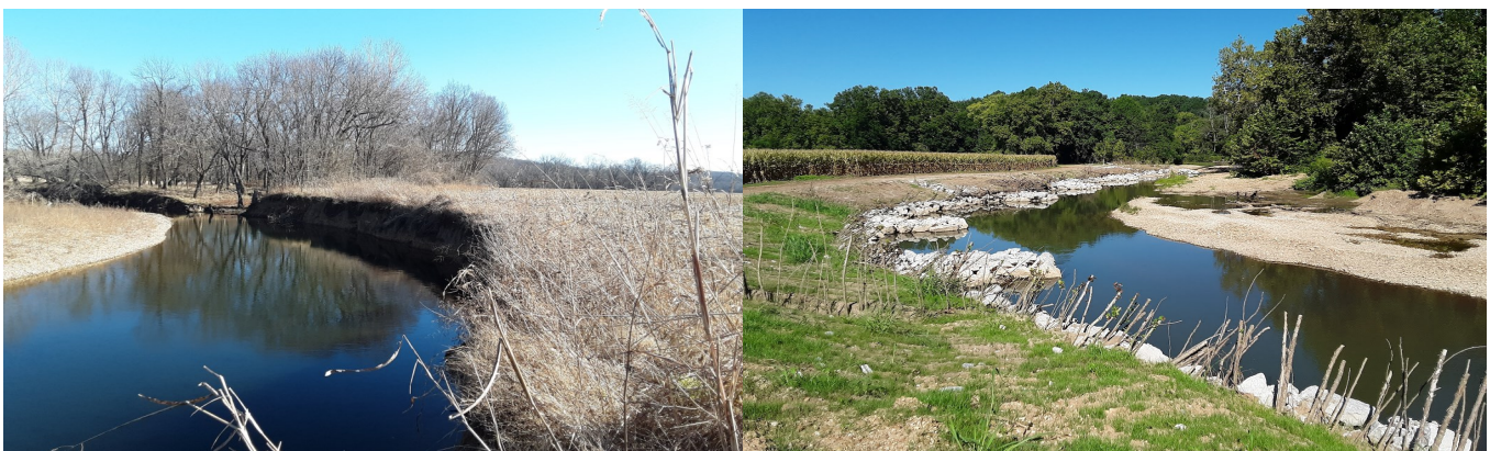
Before and after streambank stabilization on the Upper Little Sac
