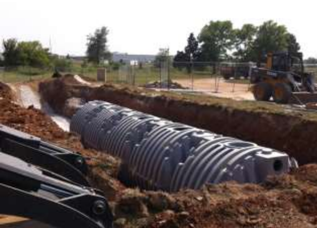
20,000 gallon rainwater harvesting system being installed at Missouri State William H. Darr School of Agriculture to provide dust suppression in arena
