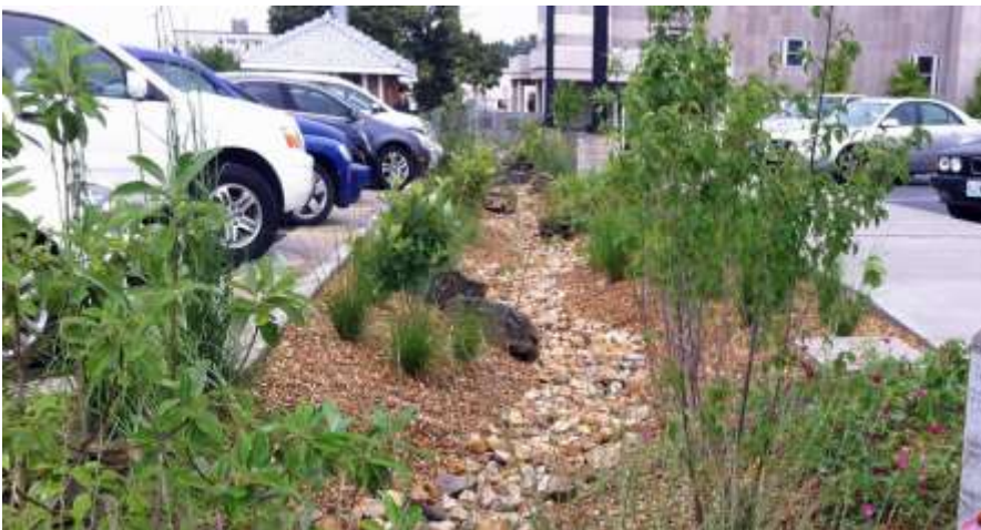
Bioswale at City Government Plaza Parking lot
