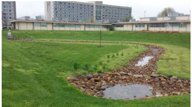
Detention basin retrofit at Missouri State University campus
