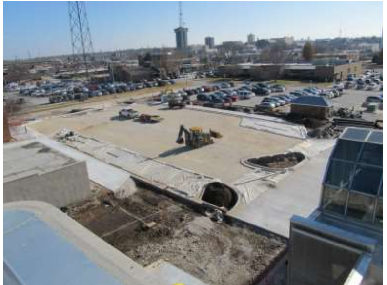
City Governmental Plaza under construction
