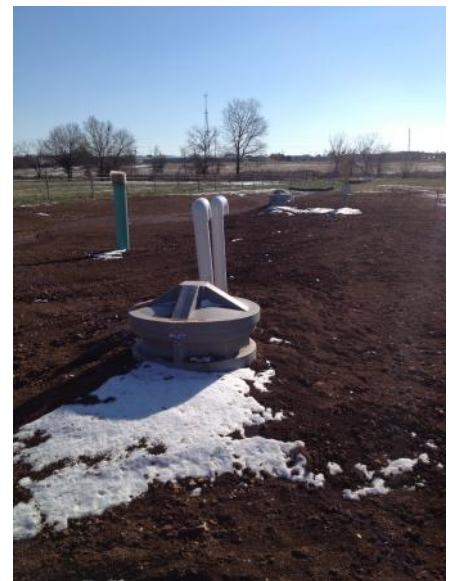
After Big Urbie Improvements
