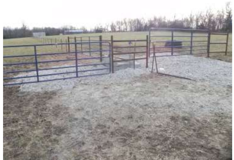
Prescribed grazing system installed including alternative watering device (center)
