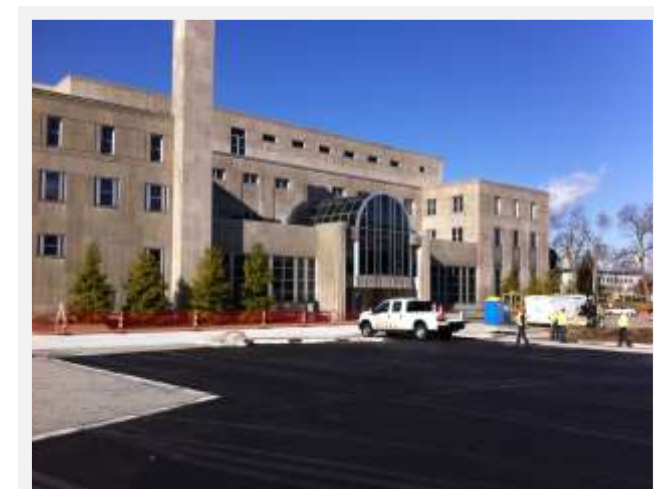
Phase 1 near completion at City Government Plaza
