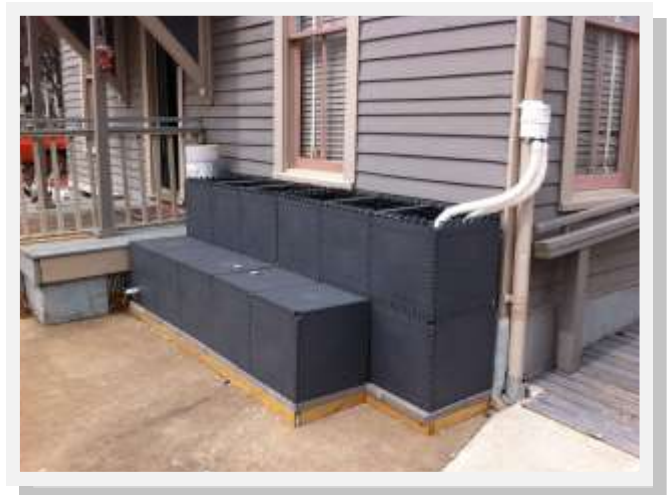
Rain water harvesting system at Gilardi's Restaurant
