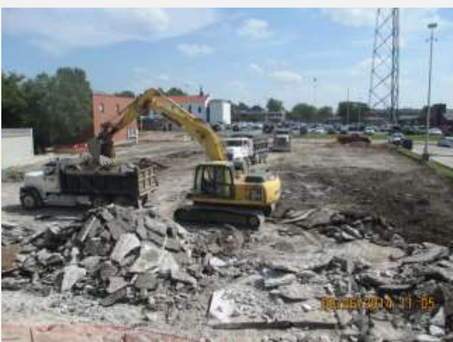
City Government Plaza, Phase 1, under construction
