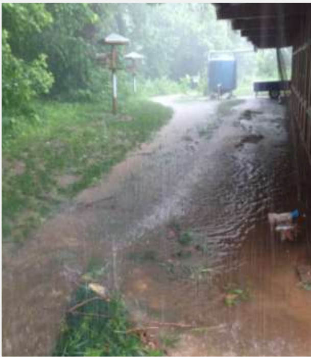
South side of C.W. Titus Education Center flooding, before site improvements
