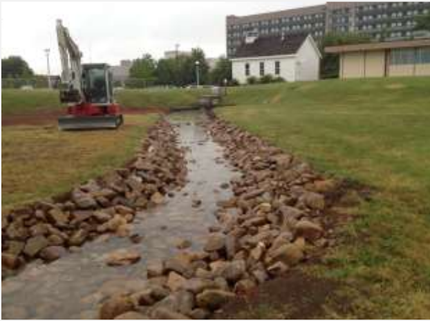
Newly constructed stormwater detention basin at Missouri State University
