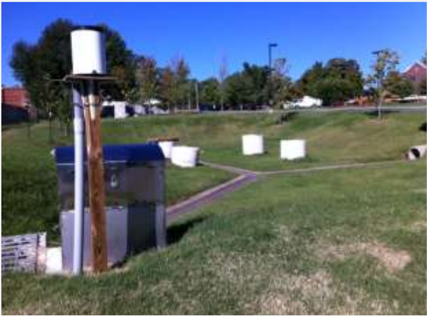
Drury detention basin will also monitor water quality
