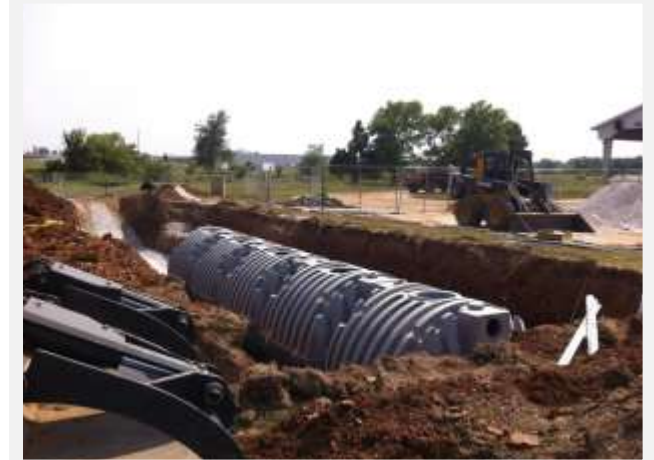
20,000 gallon rainwater collection system installation at the William H. Darr School of Agriculture
