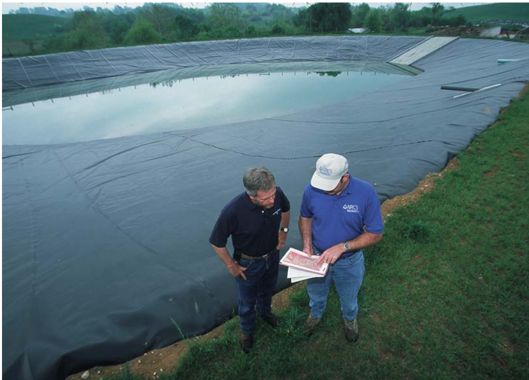
Testing the efficiency of an animal waste lagoon constructed with a preventative geotextile fabric liner.
