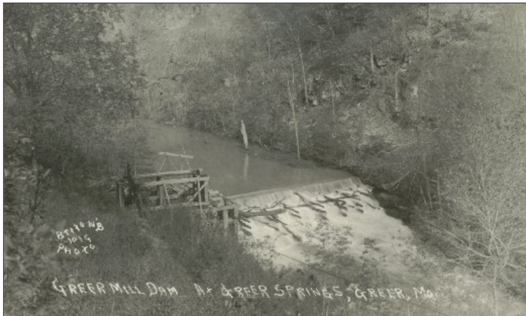
Dam and Turbine at Greer Spring
