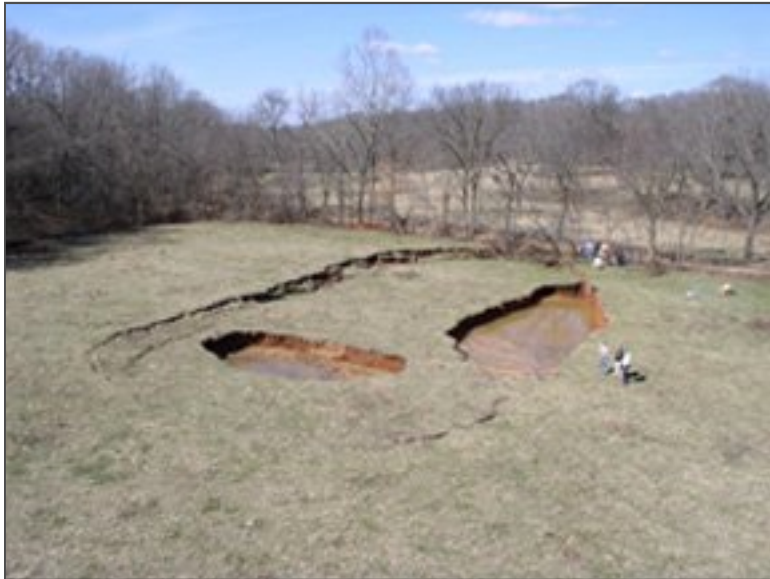
Sinkhole Collapse, Barry County
