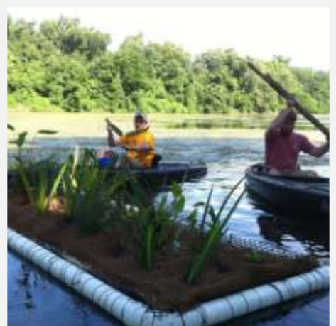
Completed Floating Wetlands being put into Valley Water Mill Lake
