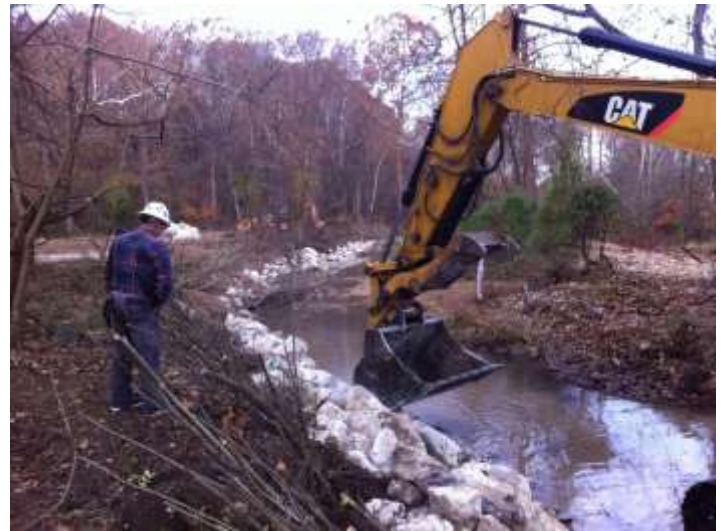
Little Sac River (downstream view) during stream restoration.
