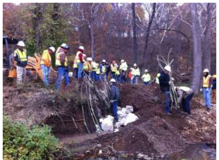
Construction of a curved key and live sycamore poles being placed.
