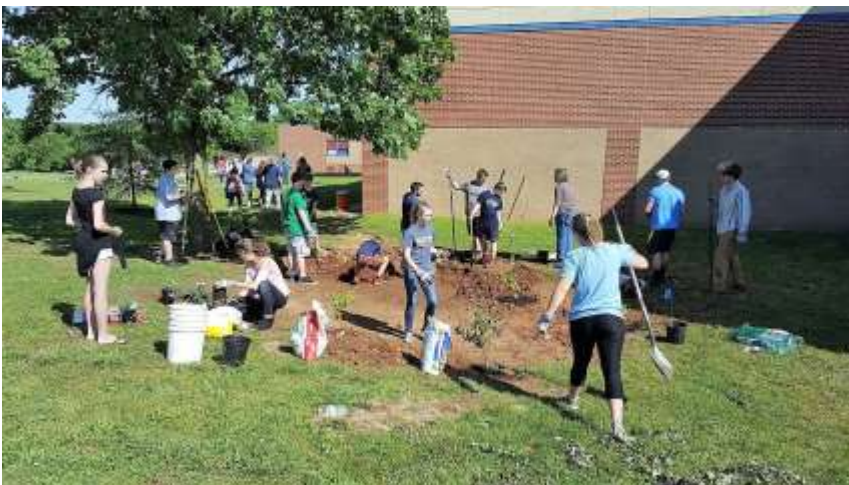
Carver students building a rain garden.
