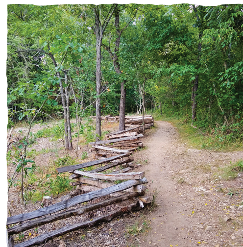
... AND AFTER WCC RESTORATION
