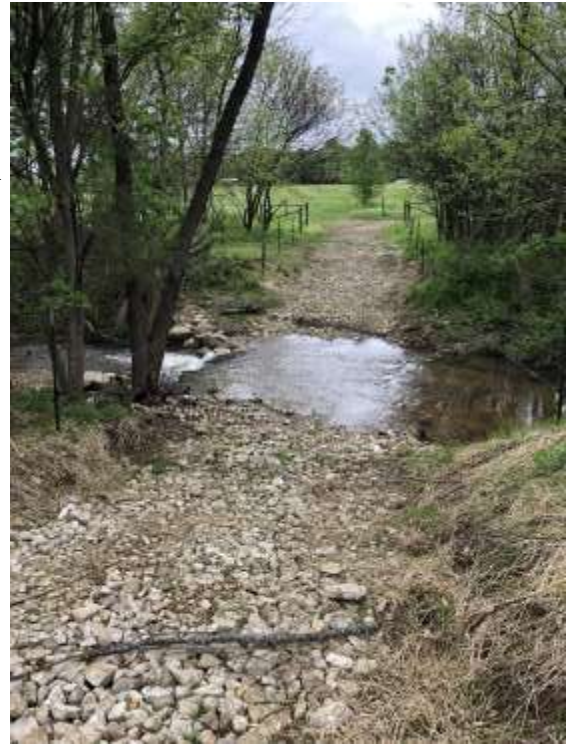
Stabilized stream crossing at the Little Sac Grazing Demonstration
