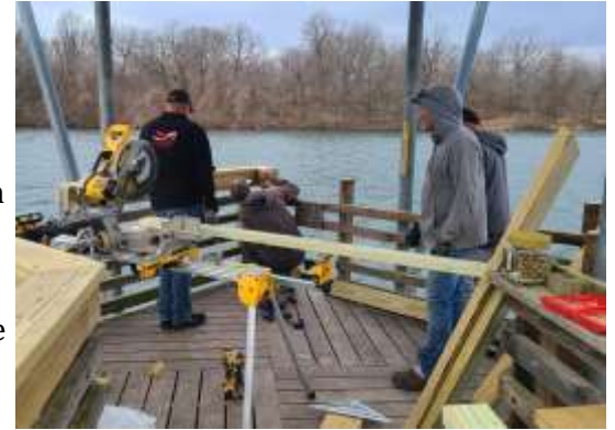
Tom and crew fixing fishing piers
