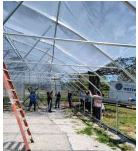
Pulling plastic poly onto the greenhouse
