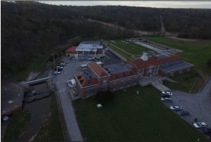
Figure 6: Fulbright Treatment Plant
