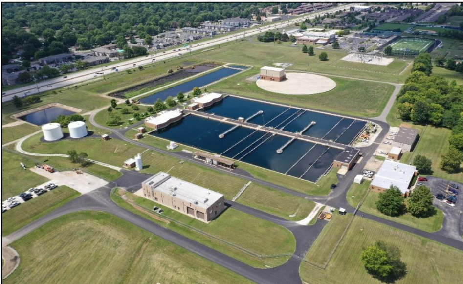
Figure 7: Blackman Water Treatment Plant
