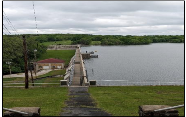
Figure 9: McDaniel Lake Pumphouse
