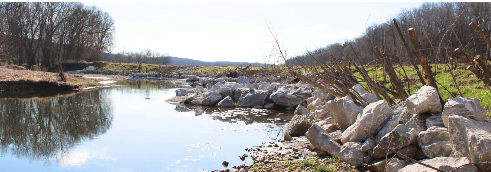
Upper Little Sac 319 stream bank stabilization
