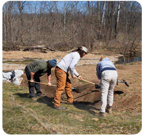
WCC and Watershed Staff Grade Ground Before Seeding
